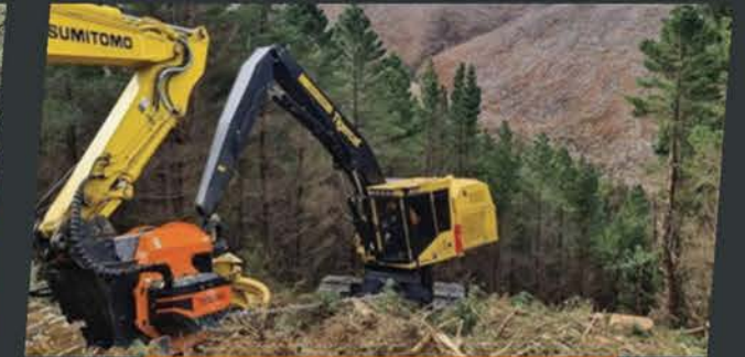
35-Ton Forestry Excavator Tethering a Feller Buncher
