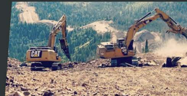
Tethering Cat 336 for Pipeline Construction
